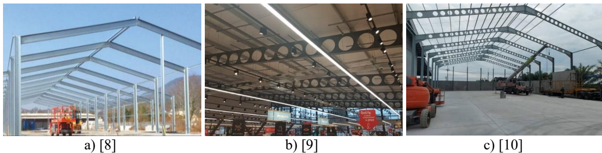
Figure 1. Elements of pitched roof systems formed by solid-web (a), single-pitched (b) and double-pitched (c) perforated steel beams.
