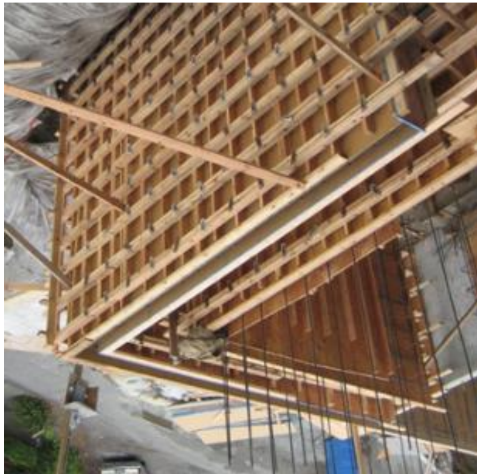
Figure 3.2 Concrete formwork
