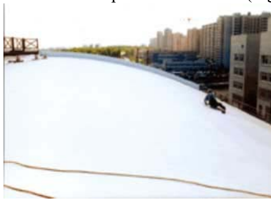
Fig. 1.2. Membrane TPO EVERGARD single-layer frost-resistant reinforced roofing membrane based on thermoplastic polyolefins
