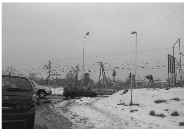
Figure 3. Railway and road crossing I.
