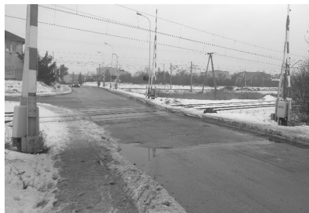
Figure 4. Railway and road crossing II.
