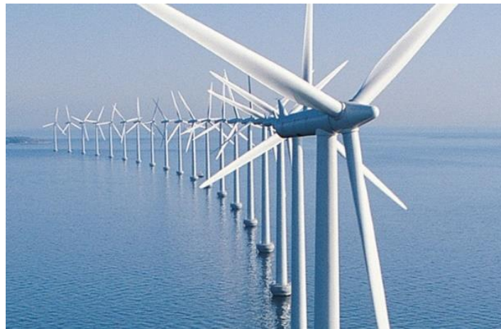
Fig. 1.6 Wind power plant
