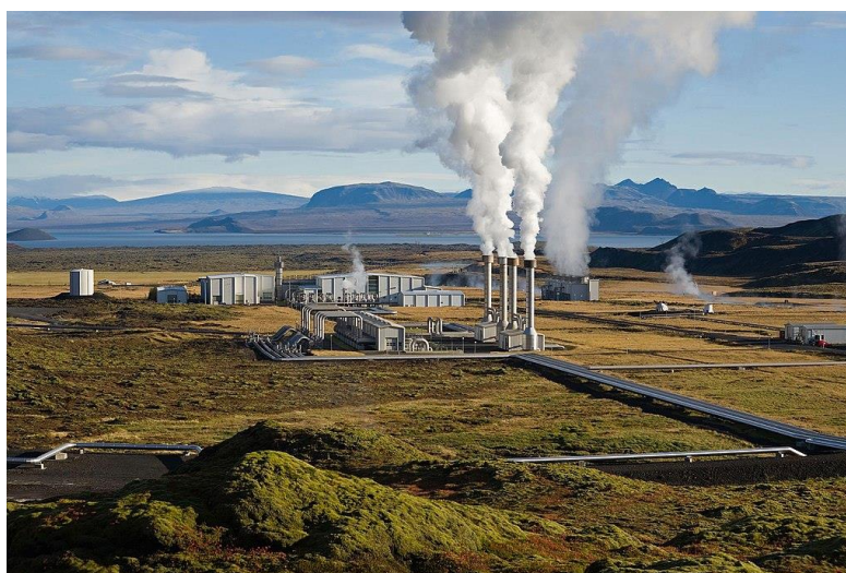
Fig. 1.10 Nesiavellir, Iceland. Geothermal thermal power plant
