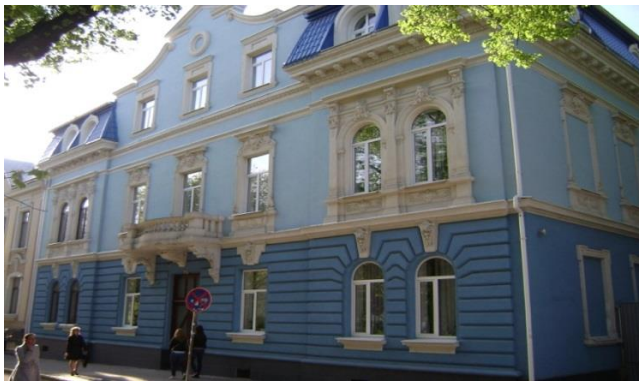
Figure 2.7 - Image of the building from the observation point 1
