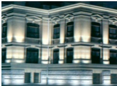
Figure 1.13 - Image of a flat view of a lighted building caused by uniform brightness of lighting perpendicular walls.
