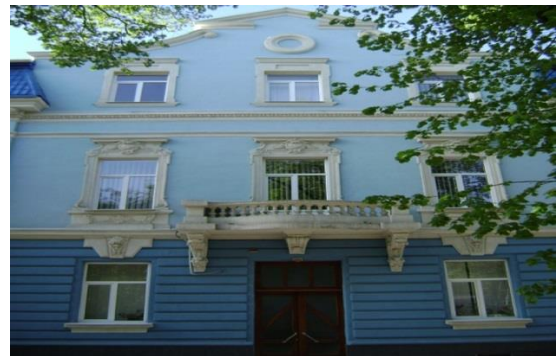
Figure 2.8 - Image of the building from the observation point 2
