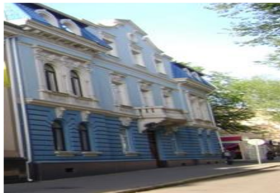
Figure 2.9 - Image of the building from the observation point 3.
