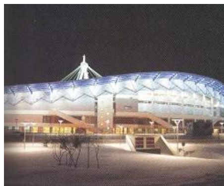
Figure 1.1 - Example of general flood lighting.
