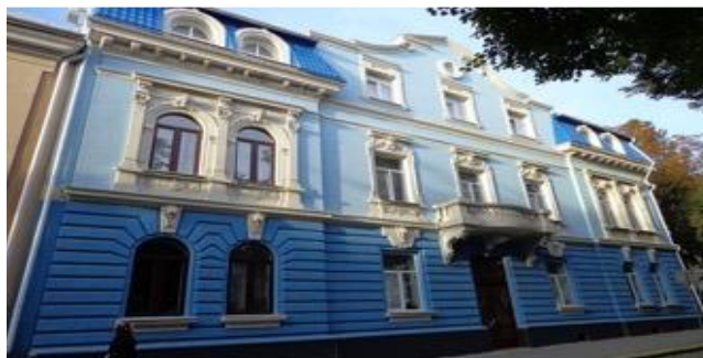
Figure 3.3 - Image of the right wing of the complex of buildings of the post office. It is located in the basement, Located on the ground floor. The second floor is occupied by department offices.
