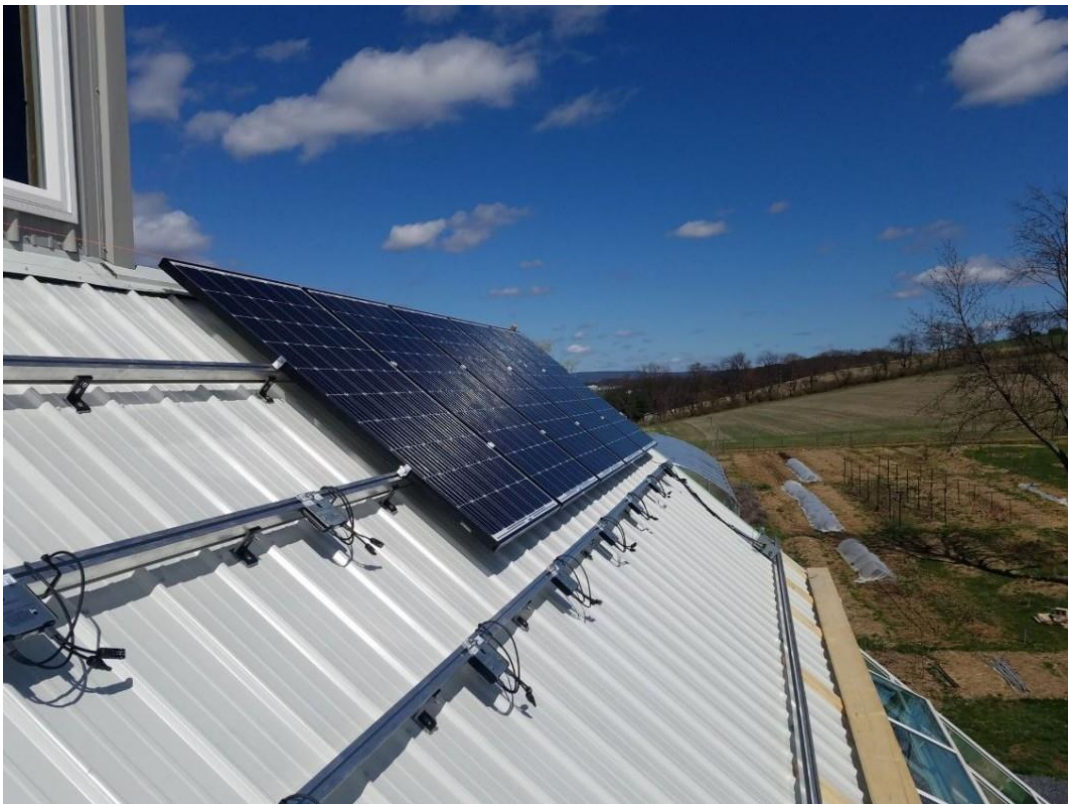
Figure 3.11. Correct installation of panels
