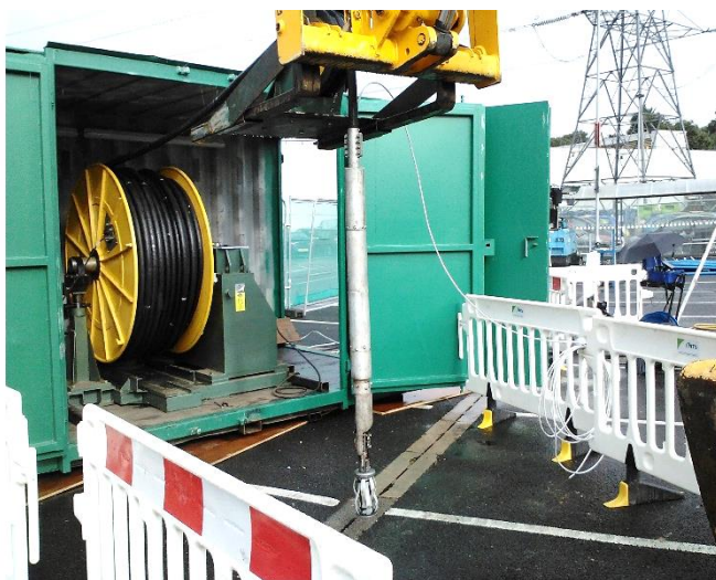
Figure 5. Installation for deep-water welding
