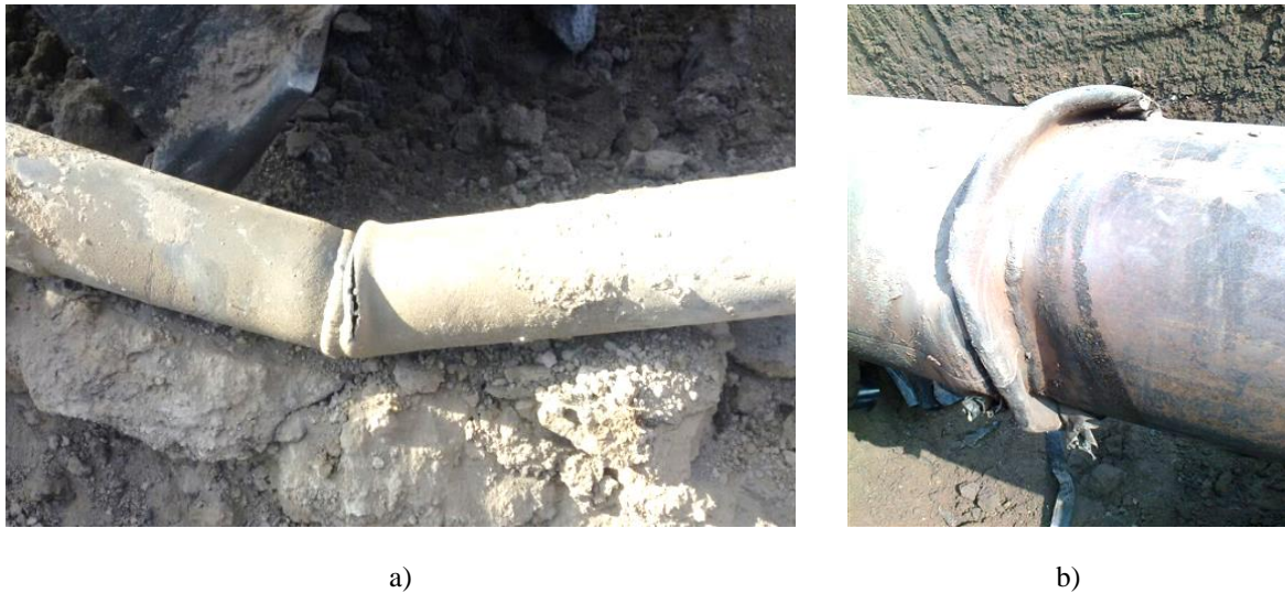
Figure 2. Examples gas pipeline failure in the surface subsidence trough: a) – DN100; b) – DN300
